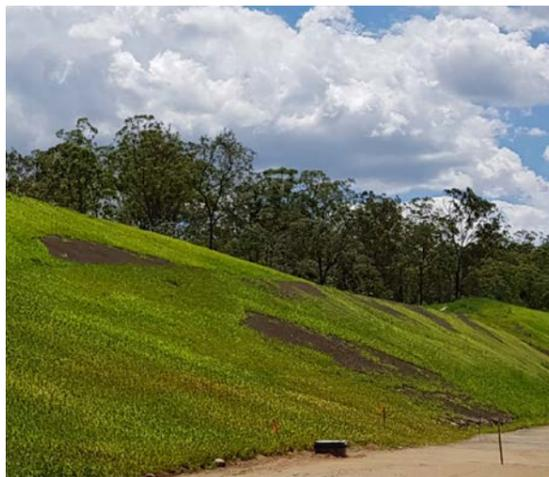
Embankments with spray grass for erosion control
