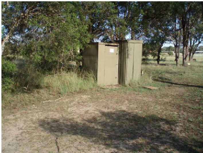
Plate 7 Shed and "toilet" located in centre of site.
