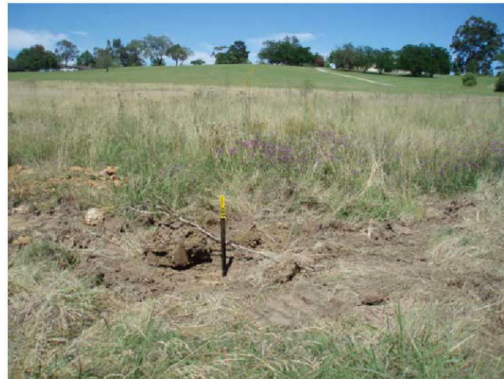
Plate 8 Location of asbestos pipe encountered at ~ 0.2. m bgl.
